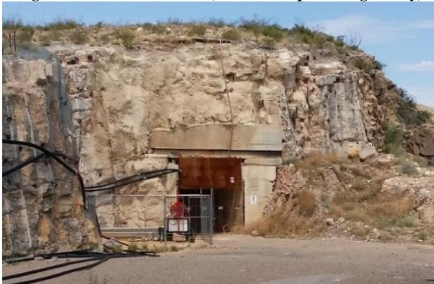
The current escape shaft (#3 Shaft) is located southwest of the office/shop/mill complex and can be used to extract miners from the mine in case of an emergency that cuts off access to the decline and Aurcana
